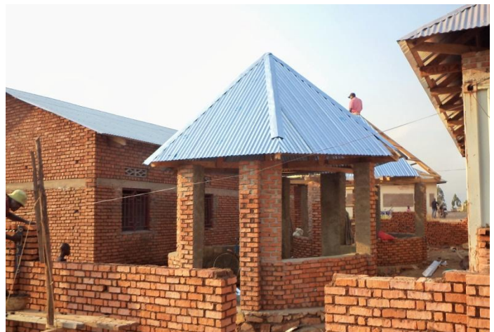
W.W. Counseling Centre under Construction.
