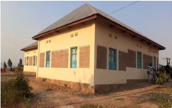
MHCD Luvungi Hospital main Building
