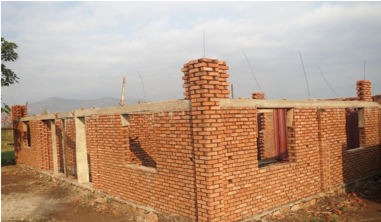
Department of Dental, Ophthalmology and Epilepsy clinic under construction.
