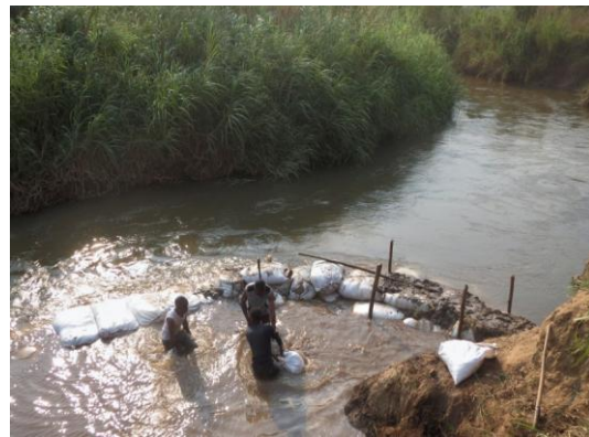
Ruvubu River where we are constructing the micro hydro power station
